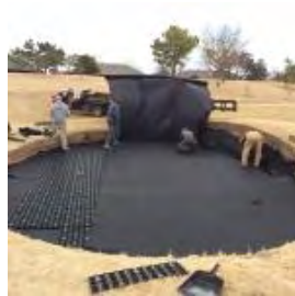
Trimming the filter fabric to fit the bunker walls.
