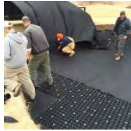
Installing the filter fabric lengthwise to minimize the seams.
