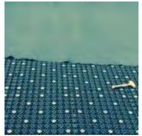
Installed with a layer of filter fabric above and below the AirDrain.
