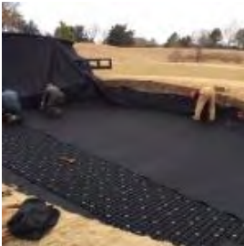
Installed with a layer of filter fabric above and below the grid.
