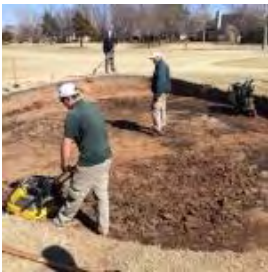
Sand removed and base prepared for AirDrain install.
