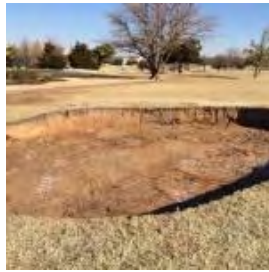
Bunker prepared for AirDrain Bunker System.
