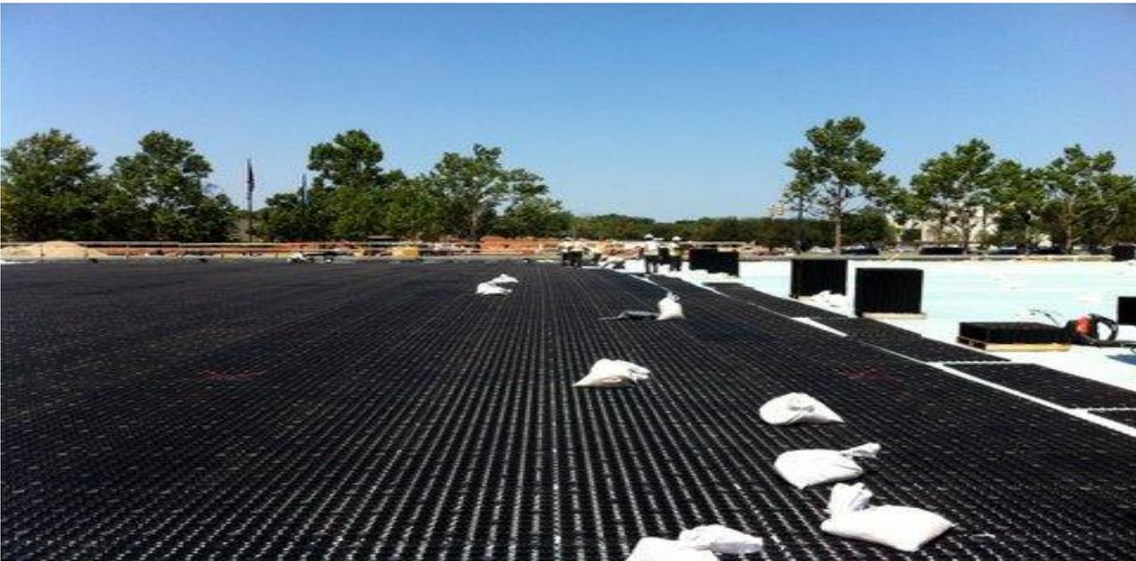
4. AirDrain panels can be shaped to individual field areas as needed with appropriate cutting device. If a typical field is installed correctly there should only be two sides that would need to be trimmed.
