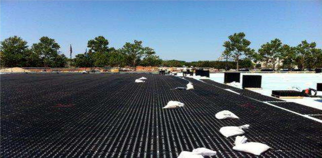
5. AirPave panels can be shaped to individual field areas as needed with appropriate cutting device.
